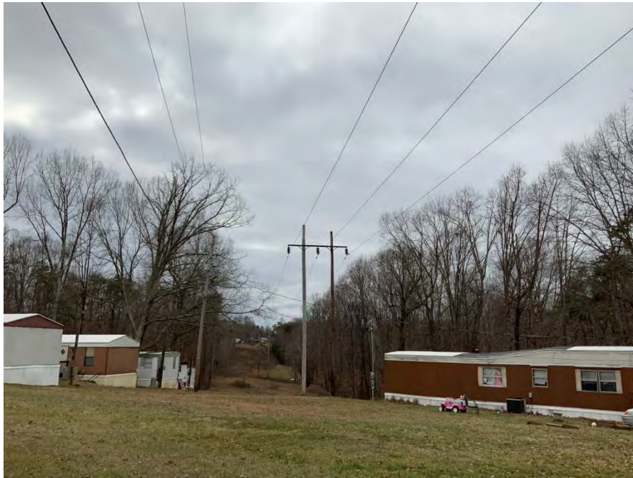
Photo 4. Existing Structure 429-49, Residential Area
