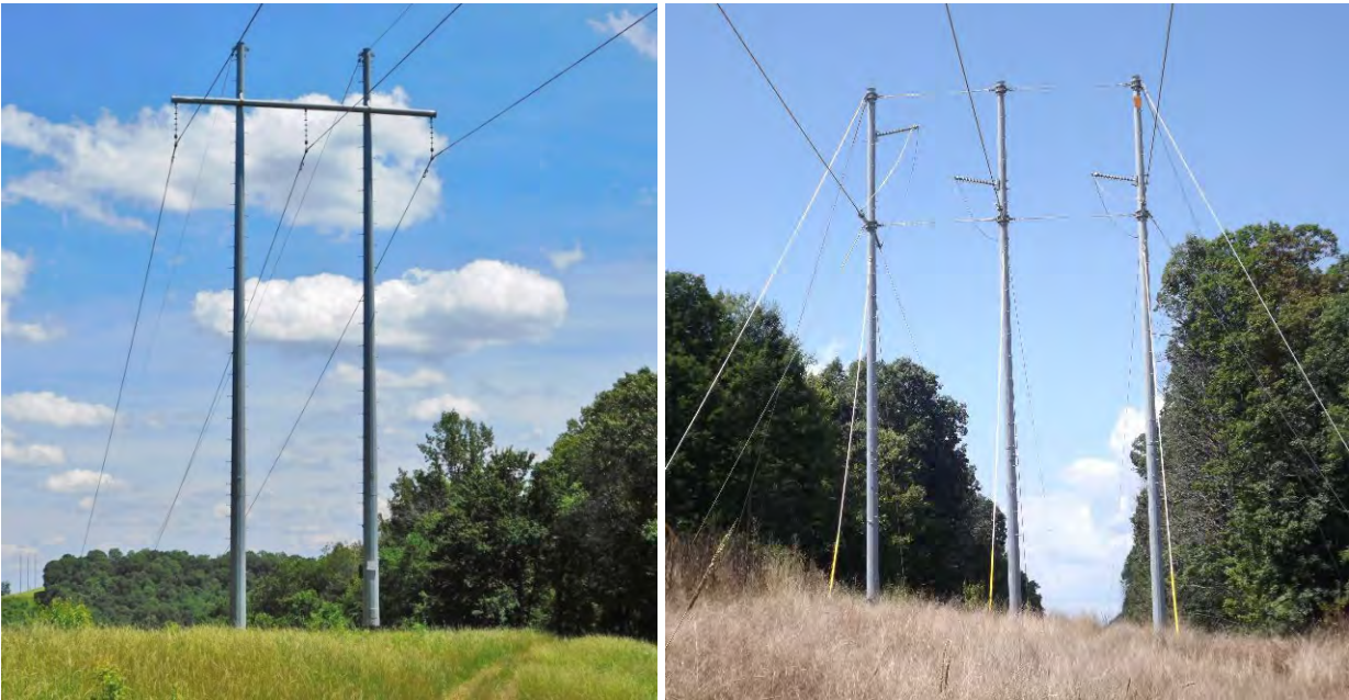
Figure 3. Typical Proposed Transmission Line Structures H-frame (left) and Three-Pole Dead End (right)
