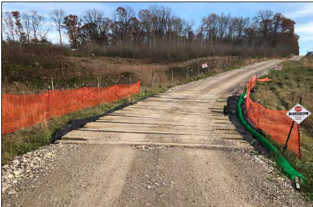
Figure 4. Typical Access Road Construction Activities
