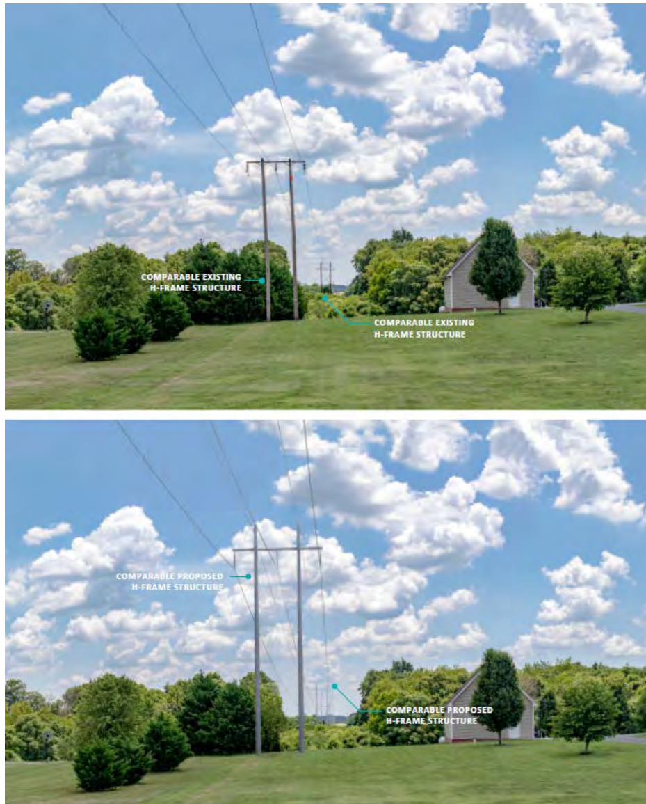
Figure 2. Comparable Existing and Proposed H-Frame Structure Existing Wood H-frame (top) and Proposed Steel H-frame (bottom)
